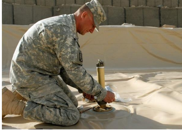
2 in. I.D. Non-collapsible Drain Hose Assembly with Bolted Flange
