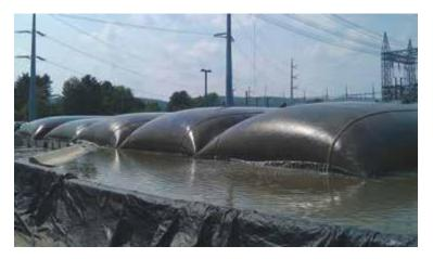
The filled geotextile tubes are stacked for dewatering in the limited lay down area.
