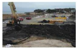
After the sediment sits and dewaters a few weeks in the geotextile tubes, the tubes are cut away. The original sediment was a marine clay and organic silt with very high water content. Without polymer treatment, it would not have been effective to dewater the materials in the geotextile tubes
