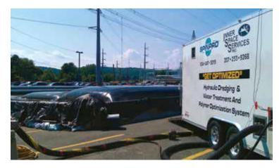
The Optimizer system trailer is where the treatment process takes place, analyzing and mixing the polymer, added to the dredge materials and then pumped to the geotextile tubes.
